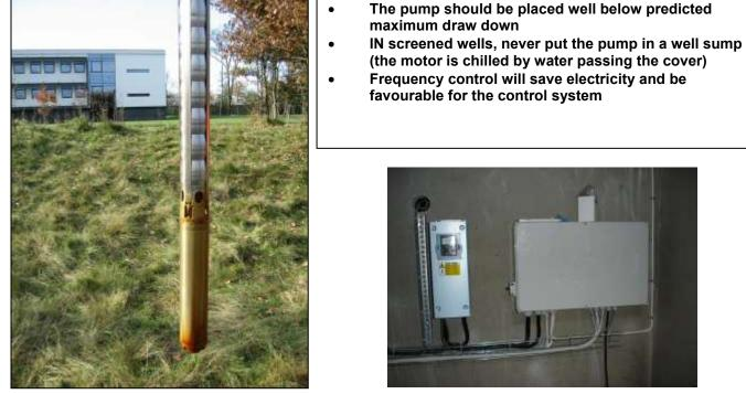
Fig.1 Submersible pump with motor and impeller and the intake of water placed between. The next image shows a box for frequency control (left) and a box for electrical connections for the pump and controlling devices in and close to the well (right).
