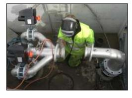
For most applications stainless steel is used for piping. However, using plastic piping is much cheaper and simpler, and corrosion resistant
