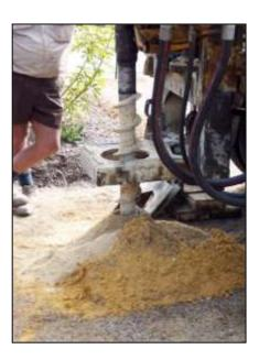
Figure 5. Auger drilling that in this case is done with hollow stem equipment.
