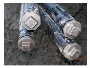
Figure 8. Example for sealing the BHE after final testing (picture: Polydynamics Engineer-
