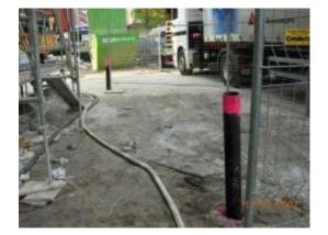
Figure 7. Protection of the BHE endings (picture: Polydynamics Engineering Zurich)
