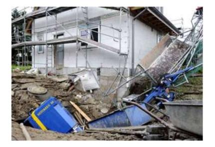
Figure 2. An undermined ground collapsed and caused damages
