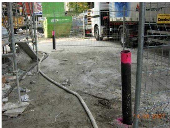
Figure 7. Protection of the BHE endings (picture: Polydynamics Engineering Zurich)
