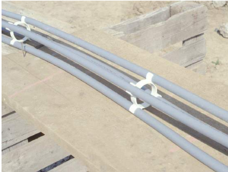
Figure 10. Double U-pipe with spacers (Neckarsulm, Germany)
