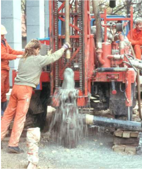
Figure 6. Artesian aquifer perforated in Hoechst (near Frankfurt); large amount of water pressing through the drill pipe
