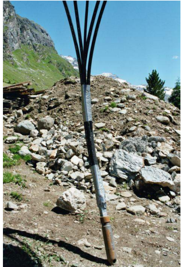
Figure 2. Ready-to-insert BHE with an additional weight, protected foot and a fifth injection tube (picture: Polydynamics Engineering Zurich)
