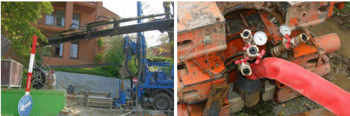
Figure 4. Guide rollers to ensure vertical insertion (picture: Polydynamics Engineering Zurich)
